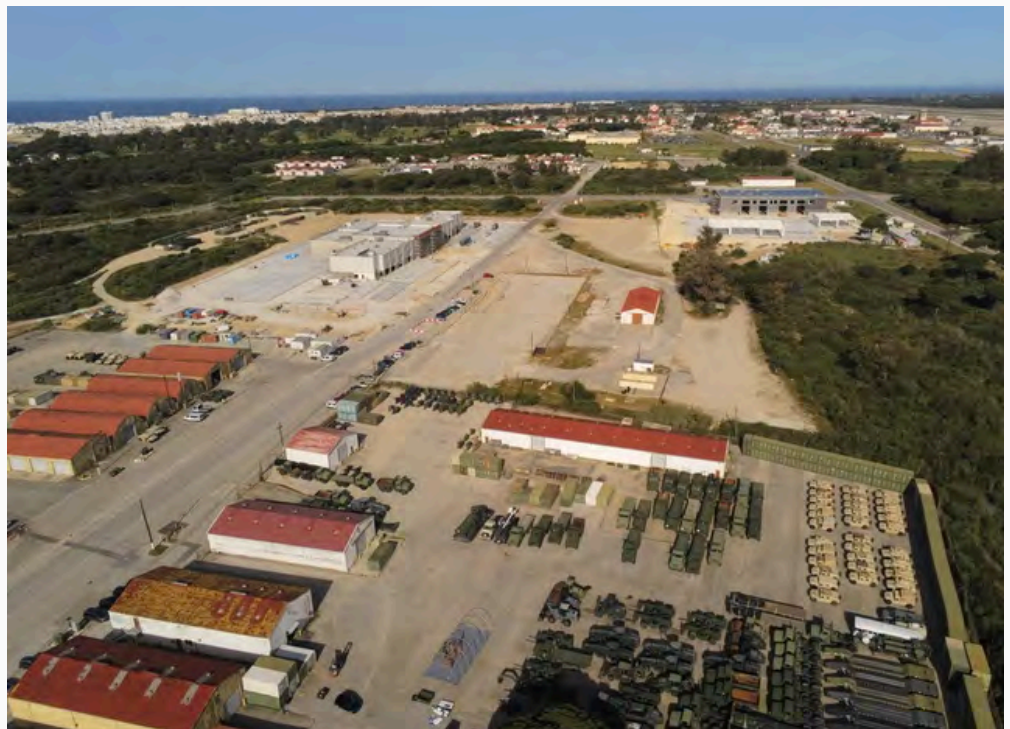
Aerial photos of Camp Mitchell at Naval Station Rota, Spain, April 24, 2025. 22nd Naval Construction Regiment commands naval construction forces for Navy Expeditionary Combat Forces Europe-Africa/Task Force 68 across the 6th Fleet area of Operations to defend U.S., allied, and partners interests. (Photo by Chief Petty Officer Justin Stumberg)
